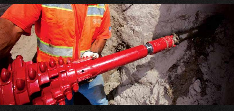
You wouldn't limit yourself to the drill bit that comes with a handheld drill. The same idea applies to your HDD tools. It's critical to only use a reamer designed to handle the specific conditions of a bore. Backreamers are the workhorse of every HDD drilling operation. For that reason, in this guide, we cover the "boring" reamer basics:
